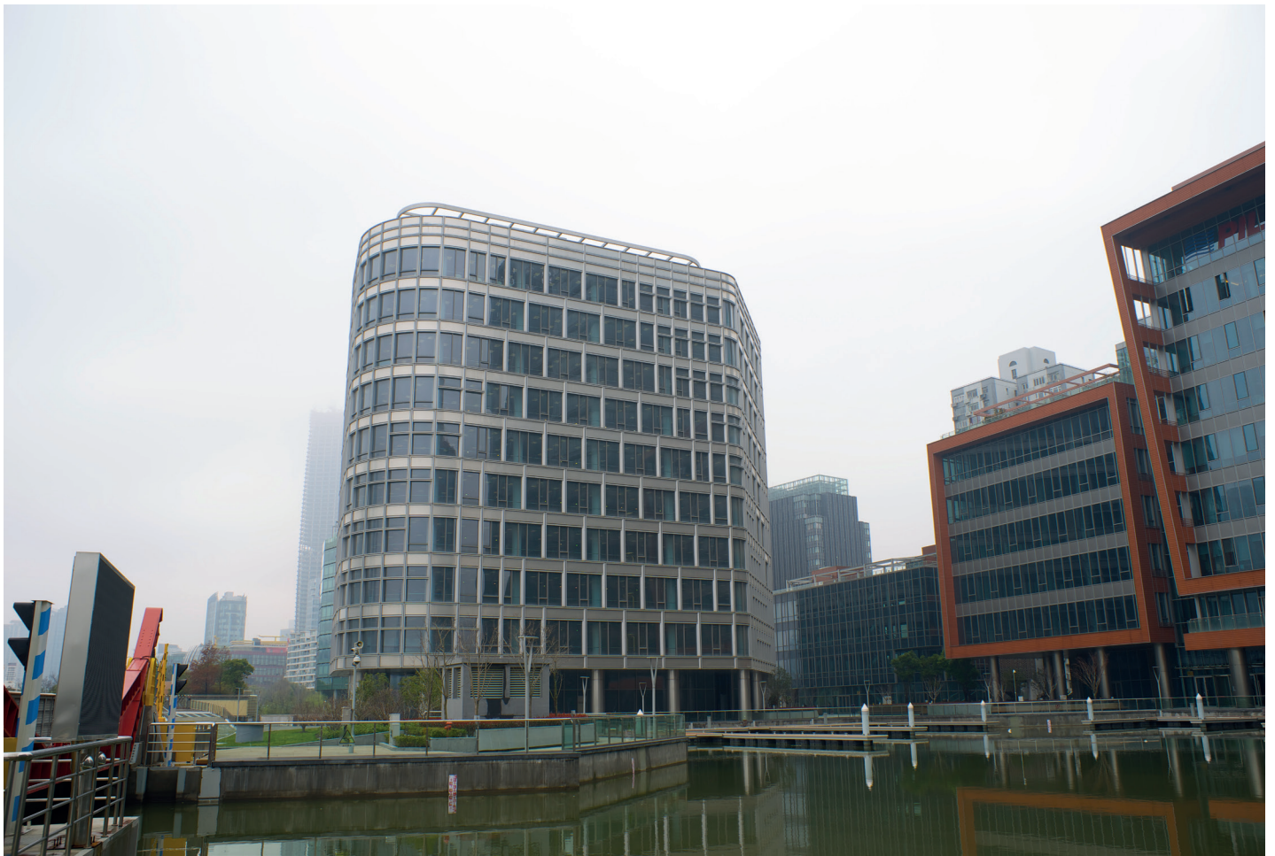
Figure 1 Harbour side view of Building 17, 17号楼港口侧外观
