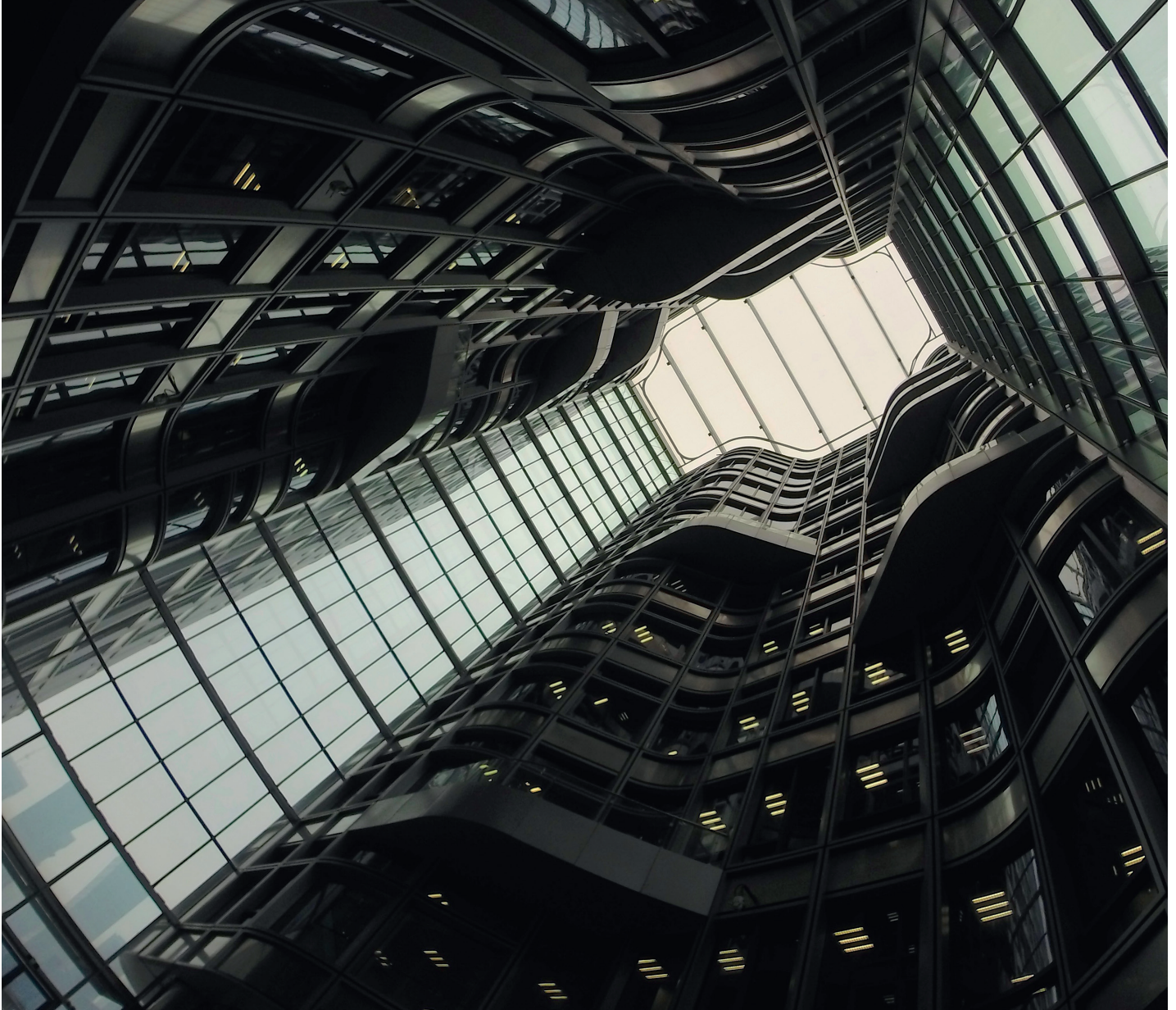
Figure 2 Atrium of building 17 17号楼中庭
